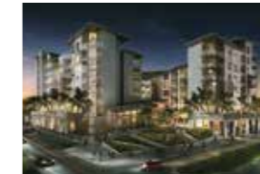
Panama Mosaic Building PANAMA PACIFICO
